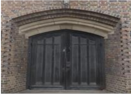
Retain and protect the main doorway from Old Oak Road
