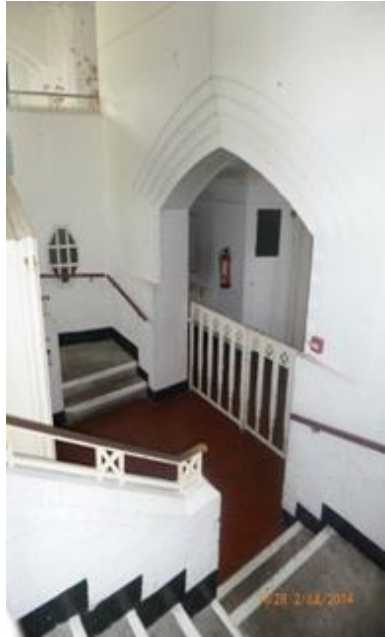
Retain and protect the feature twin stairs and the iron gate
