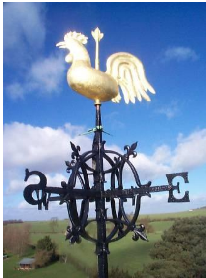
The restored weathervane on the Tower
