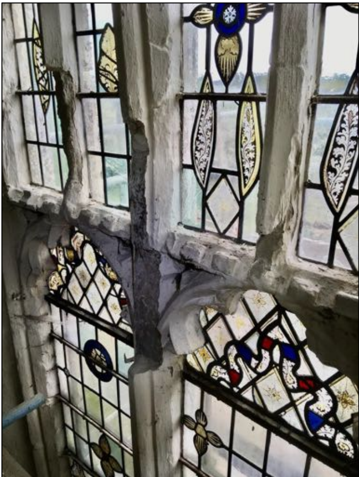
Investigations revealing the poor condition of the east window, and the stress it was putting on the medieval glass
