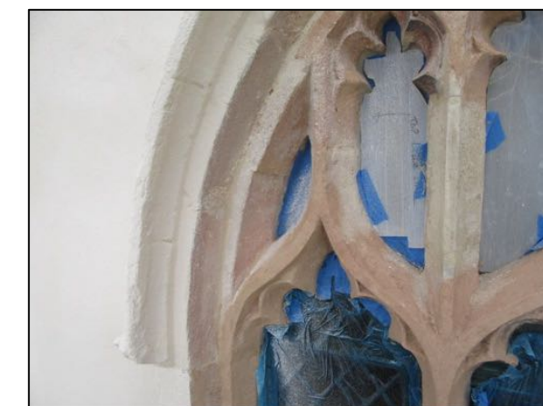
Conservation of window masonry in progress, by Gem Conservation before shelter coating
