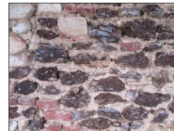
Condition of rubble walling once cement pointing was removed revealing many cavities allowing water to pass deep into the wall, saturating the masonry, and without being able to dry out effectively
