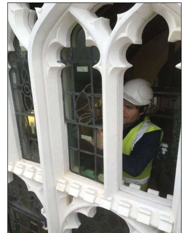
Specialist glazier, Devlin Plummer, reinstating the glass to the east window
