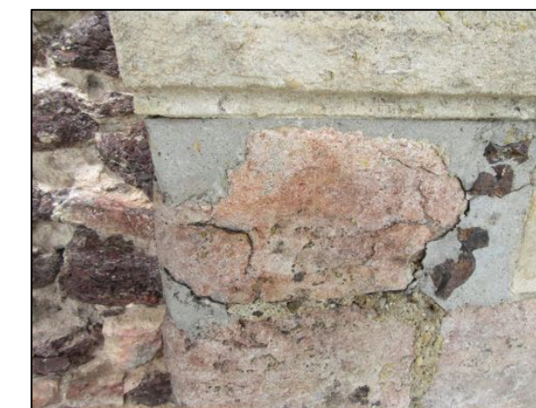
Poor condition generally of chancel windows and buttress dressing following cleaning, showing multiple fractures, loss of details, previous cement repairs and erosion from lichens and weather
