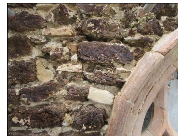
Condition of rubble walling once cement pointing was removed revealing many cavities allowing water to pass deep into the wall, saturating the masonry, and without being able to dry out effectively
