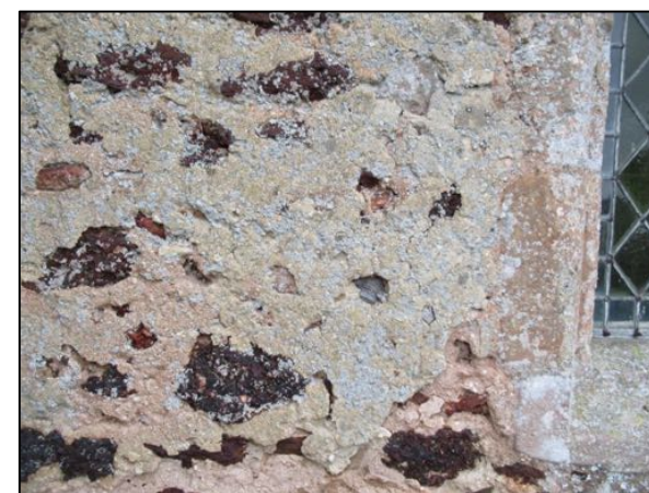
Existing evidence of render base coats with exposed porous rubble walling, all covered in lichen adding to inexorable decay
