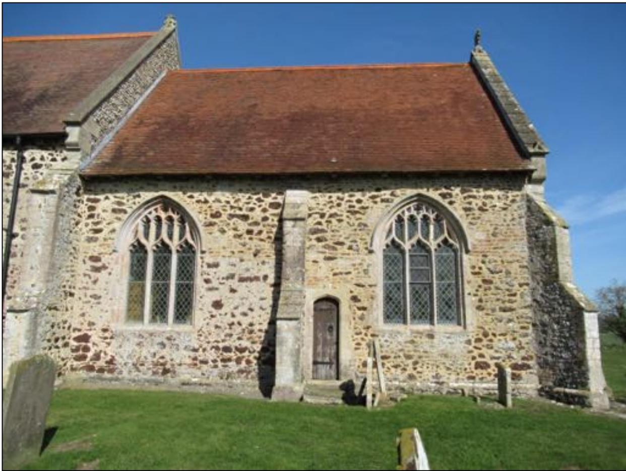
Chancel - south elevation, showing extensive cement pointing to the rubble walling
