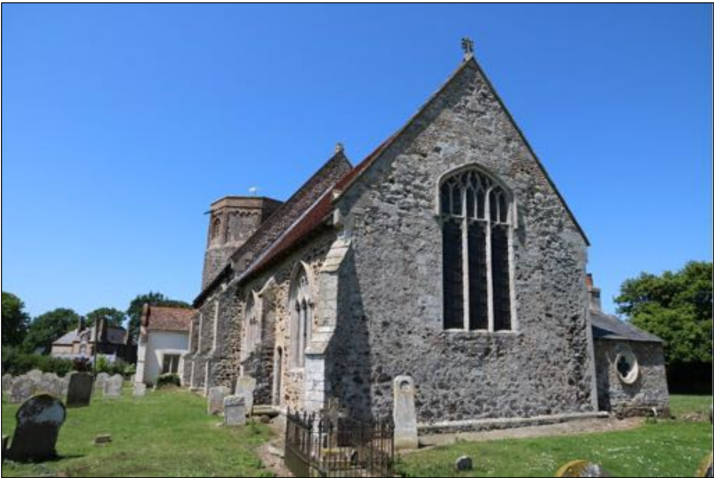
Chancel - east elevation, showing remnants of render and a lot of C19 brick replacement to the gable
