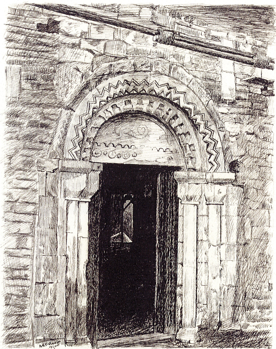
S outh doorway, drawn after removal of porch during restoration For description see page 73.
